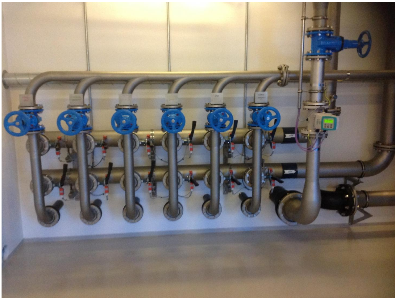
Figur 1: Fordelingsarrangent for råvand, kaldet vandorglet.
