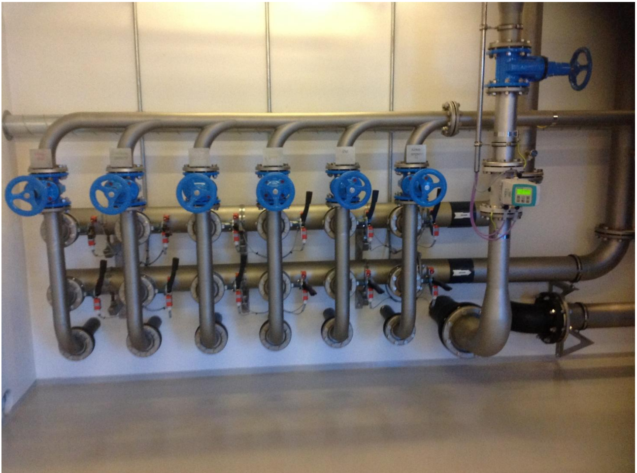
Figur 1: Fordelingsarrangent for råvand, kaldet vandorglet.
