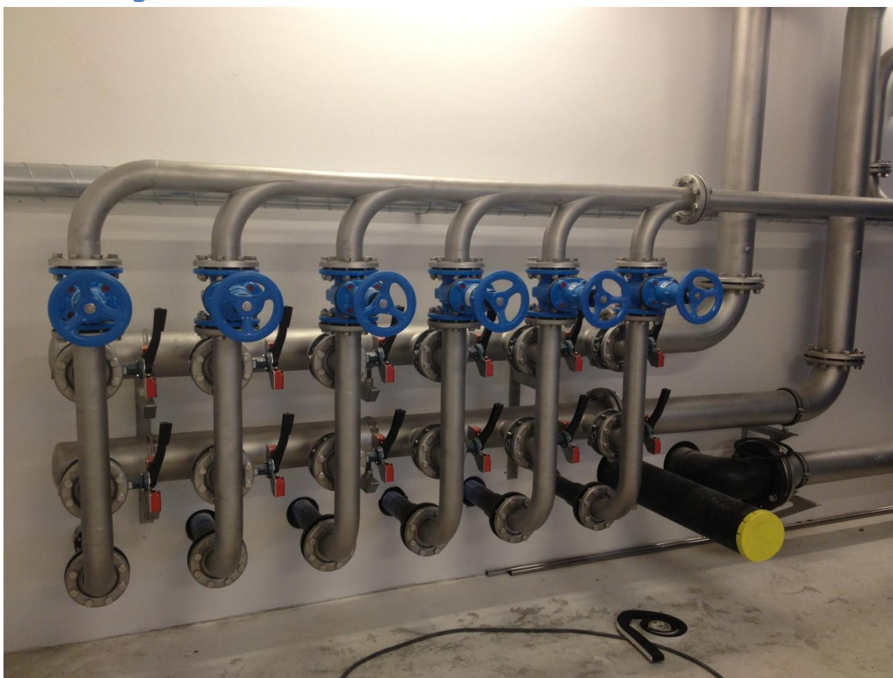
Figur 1: Fordelingsarrangent for råvand, kaldet vandorglet.
